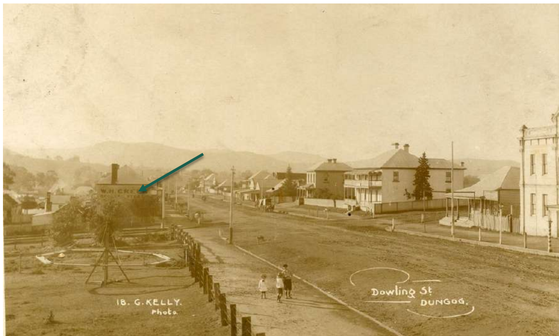
Figure 5 Dowling St. Dungog. 18. G. Kelly. Photo [1908] source: Living Histories
